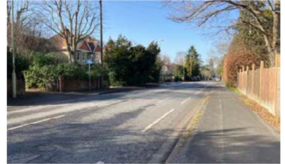
Narrow existing cycling facilities along Kings Road
