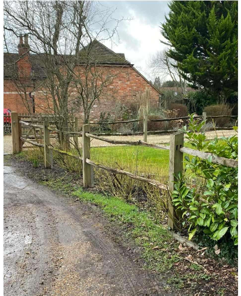
Timber post-and-rail fencing at No. 1 Handcroft Cottage, Pankridge Street
