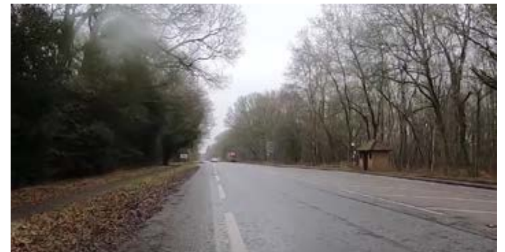
A30/London Road near The Hogget bus stop
