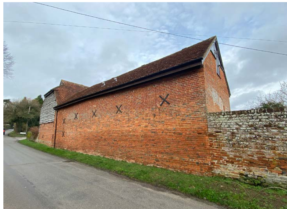
Hannam's Farm Barn, Itchell Lane
