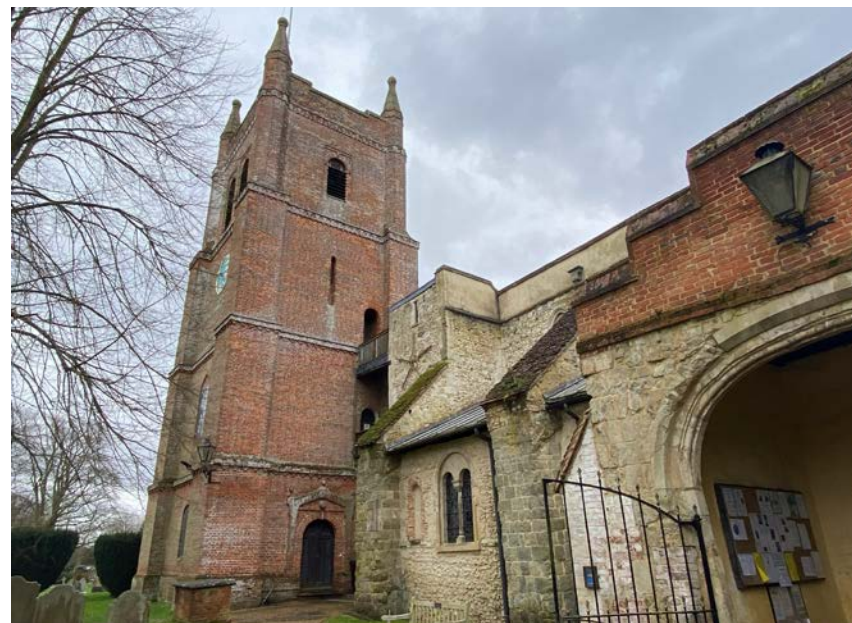
North elevation of All Saints' Church
