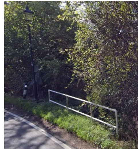
The utilitarian balustrade to the River Hart on Crondall Road with an adjacent “Windsor” style heritage lamp
