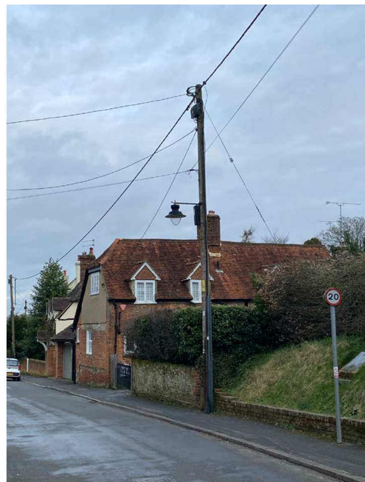
Telephone poles and overhead wires on Church Street
