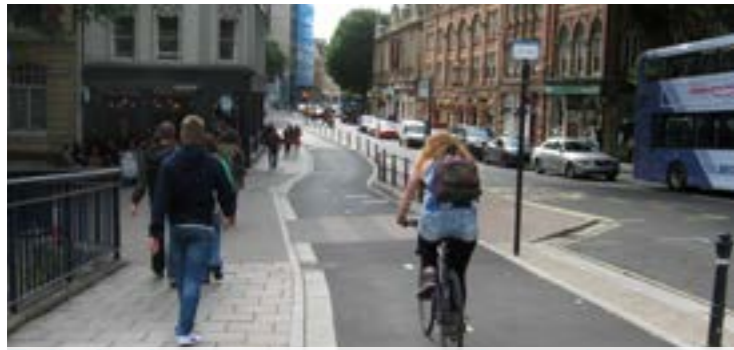
Fully kerbed segregated cycle track
