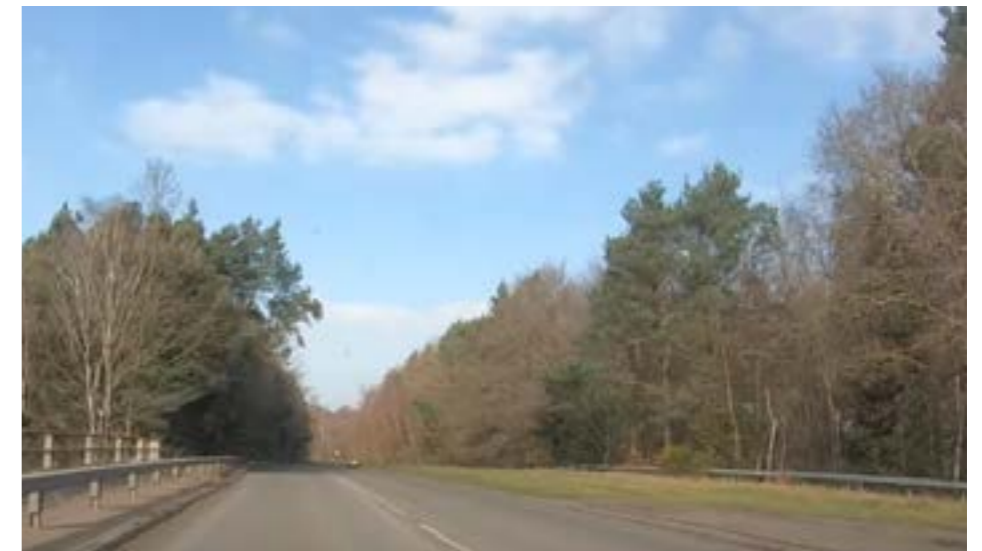
Minley Road M3 overpass
