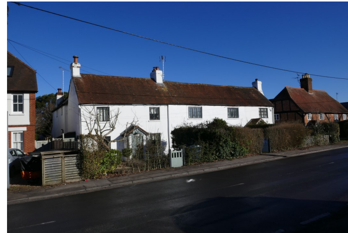
Stretch of soft hedging to the north of Crossways
