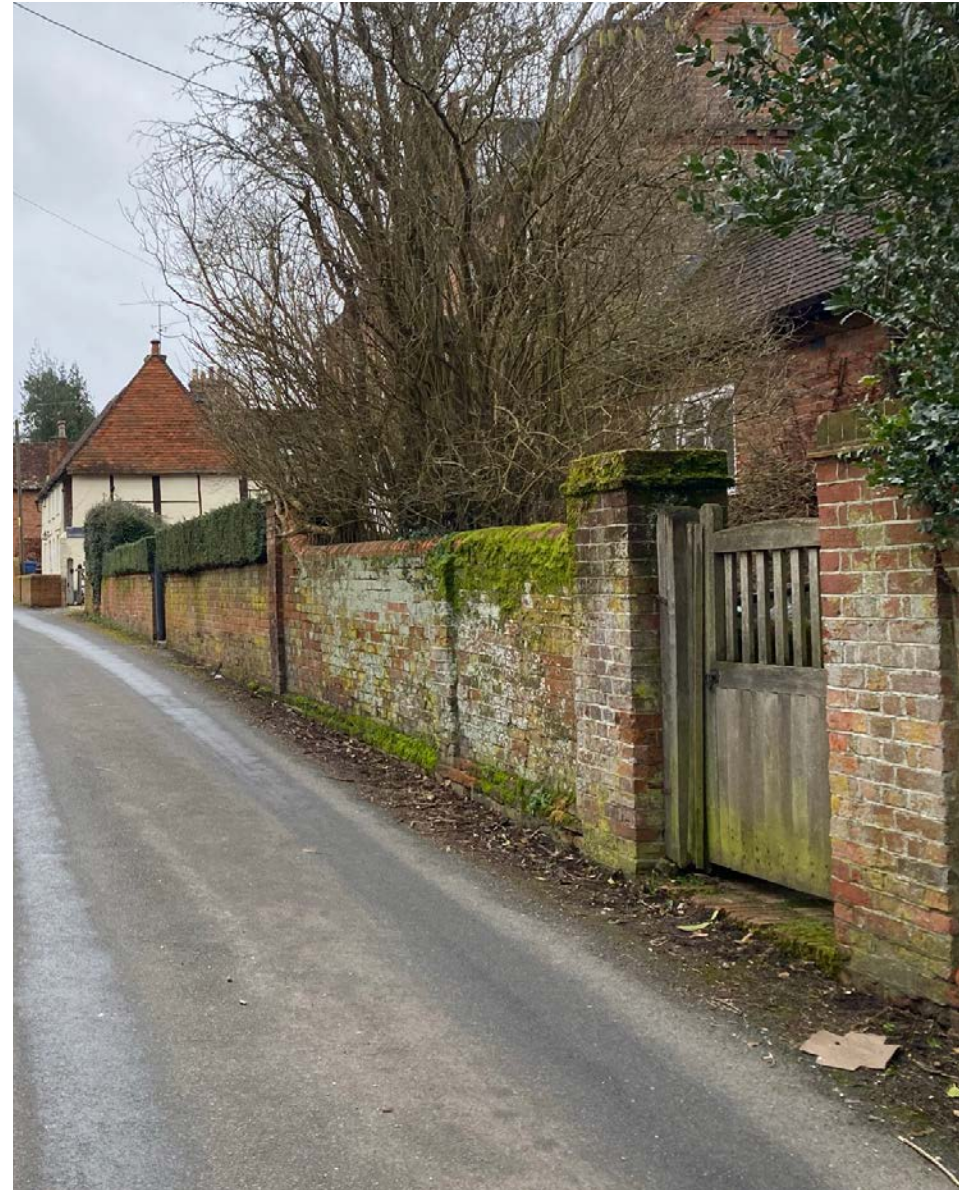
Brick boundary walls on Church Street
